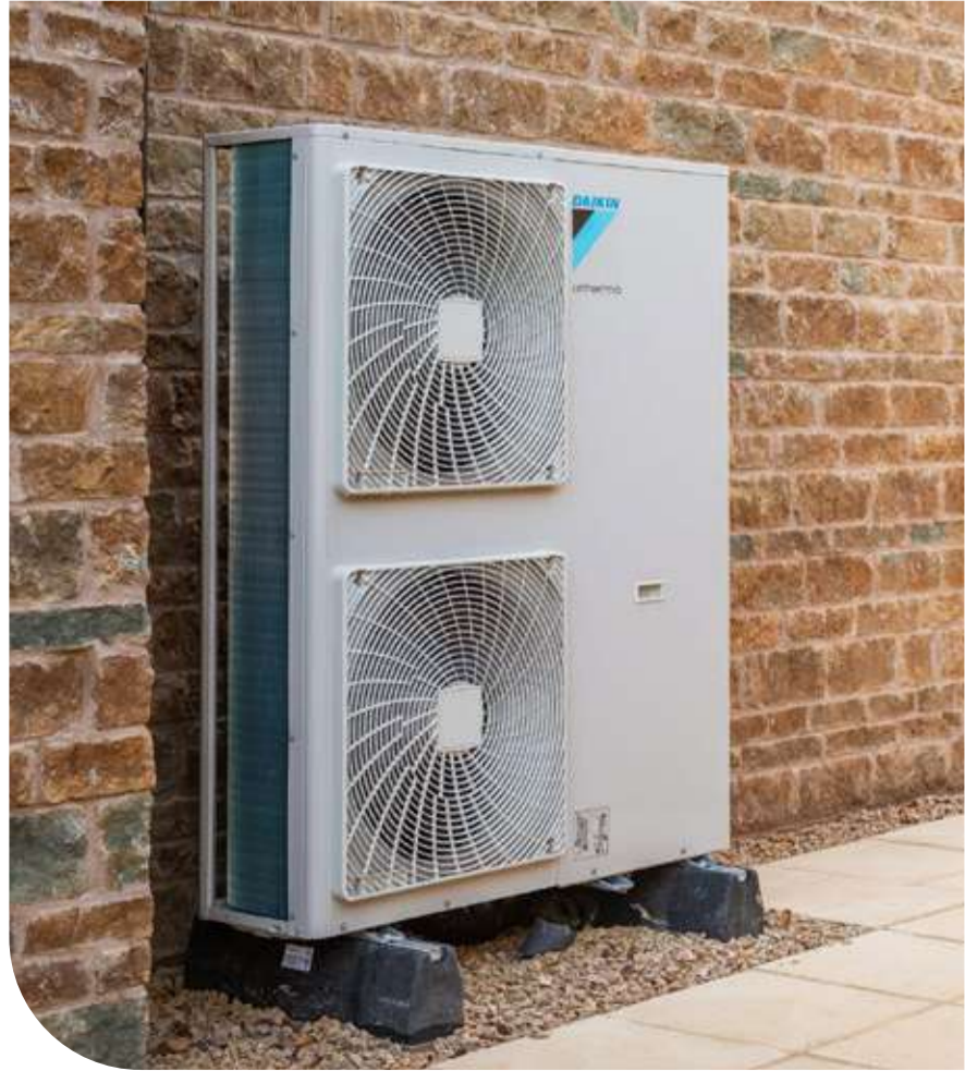
Figure 3.5: Air source heat pump.
