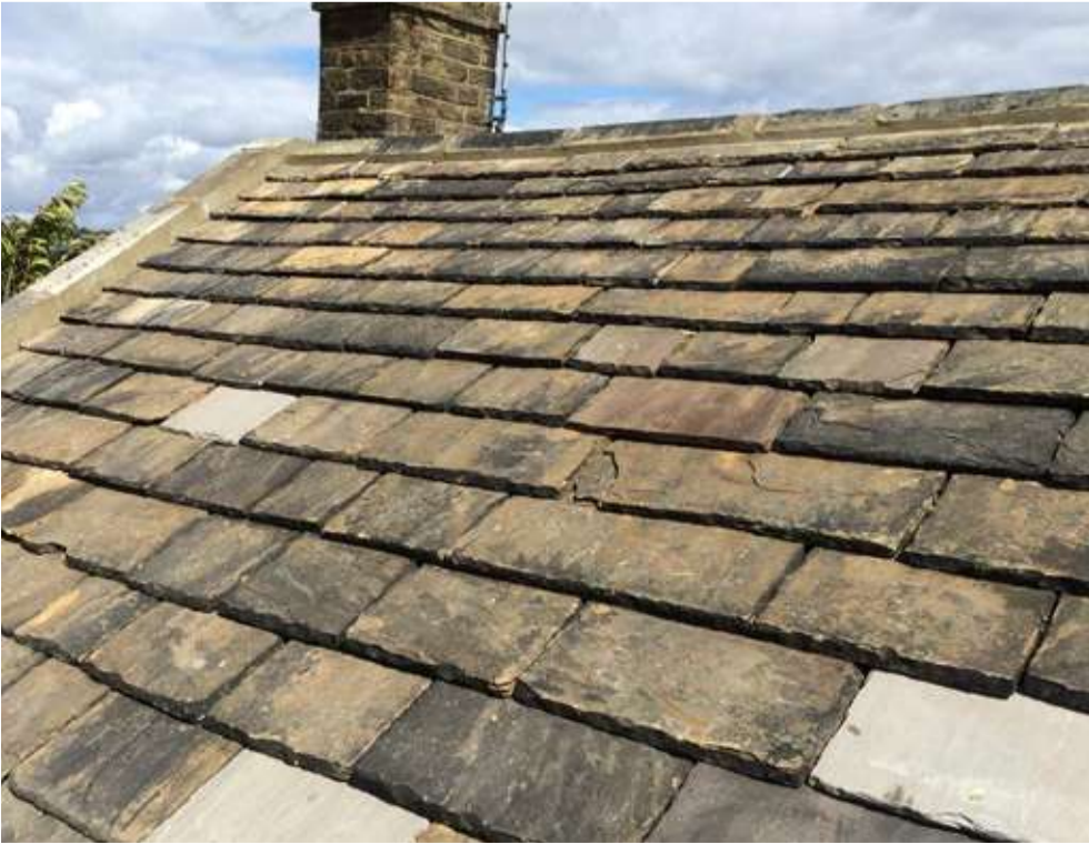
Figure 2.2: Stone slate roof with stone chimney.
