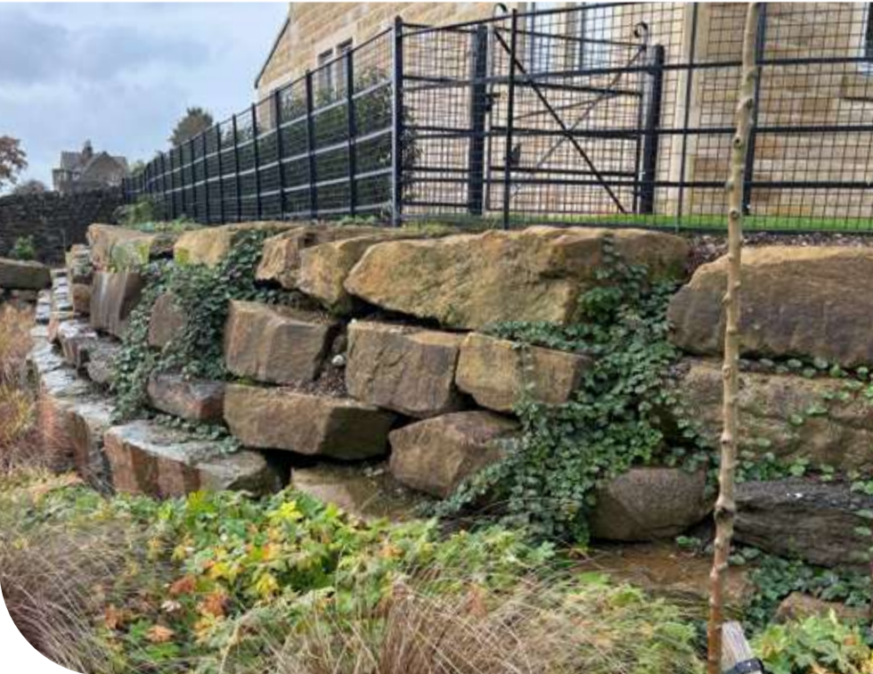
Figure 1.1: Boulder retaining wall with planting and estate railings.
