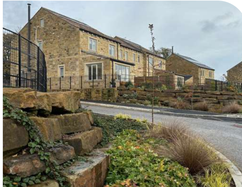
Figure 1.6: Boulder retaining wall with native tree and shrub planting.
