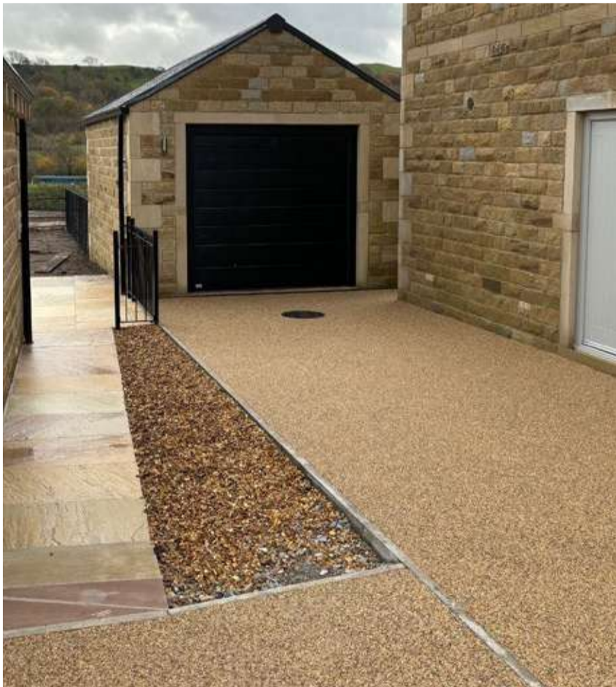
Figure 3.3: Permeable surface - resin bound driveways.
